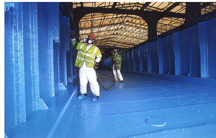
Figure II – Anderton Boat Lift, UK
