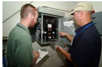
Above: Jeremy Hailey (right), a NACE International cathodic protection (CP) course instructor, demonstrates how to test a CP system during a CP-1 course field training on Sept. 21 at Bolling Air Force Base, Washington D.C., in cooperation with the 11 th Civil Engineer Squadron. CP helps engineers prevent the corrosion of underground pipes. The level-1 training course is provided by NACE in cooperation with the DoD to train system technicians. U.S. Air Force photo courtesy of Staff Sgt. Amber Whittington.
