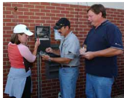
Above: Charles Henderson (center), a NACE International cathodic protection (CP) system course instructor, shows students how to test a CP system during a course field training conducted at Bolling Air Force Base, Washington D.C., on Sept. 21, in cooperation with the 11 th Civil Engineer Squadron. U.S. Air Force photo courtesy of Staff Sgt. Amber Whittington.
