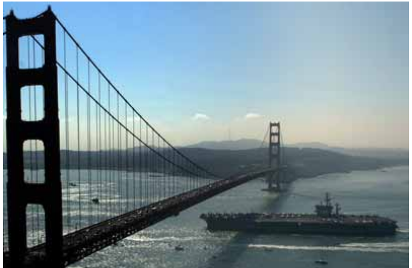
The aircraft carrier USS Nimitz passes under the Golden Gate Bridge while entering San Francisco Bay during San Francisco Fleet Week 2006. NAVSEA is solving one of the most serious aircraft carrier corrosion problems that exists today. U.S. Navy photo by Mass Communication Specialist 2nd Class Charlemagne Obana.
