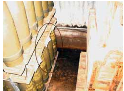
Ammunition shows corrosion inside the storage facility at Fort A.P. Hill. Photo courtesy of Army Corps of Engineers.
