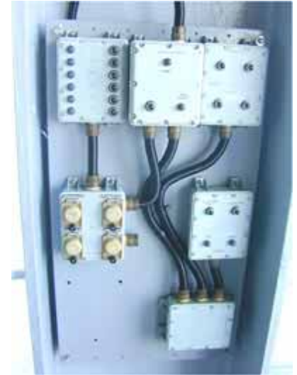
The new composite electrical box is expected to have a lifetime of 30 years and avoid millions of dollars in man-hours, repair, and replacement. Photo courtesy of NAVSEA.
