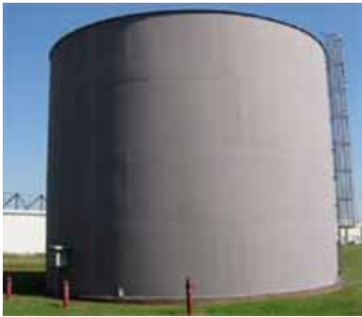
A deluge tank at Fort Campbell, situated across the Tennessee/Kentucky border and home to the 101st Airborne Division, has benefited from the Corps of Engineers' patented self-healing coating. Photo courtesy of Army Corps of Engineers (CERL).
